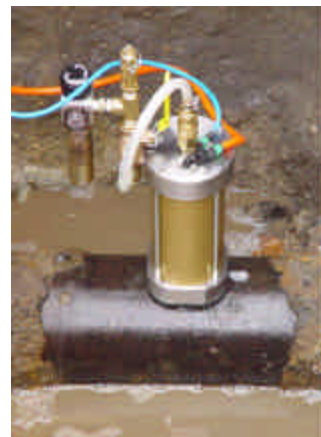
Figure 16 : Functional pre-prototype unit installed in a live cast-iron gas main
